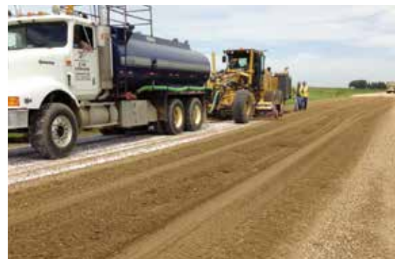
Dry calcium application.
